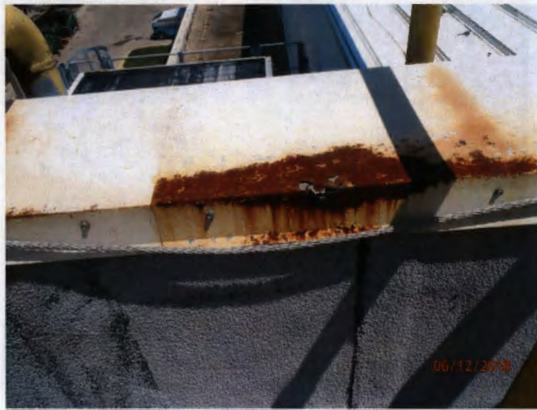
CORRODED PARAPET CAP
