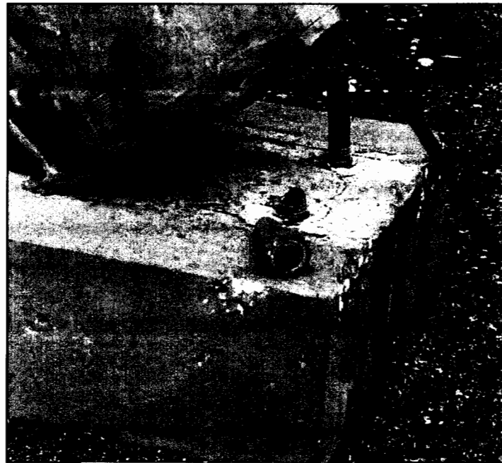
Figure 18: Building 9, Fracture of anchor bolt
