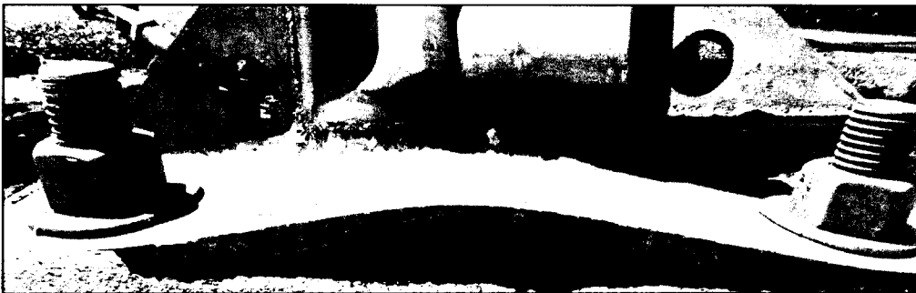
Figure 5: Building 1, Yielding of baseplate
