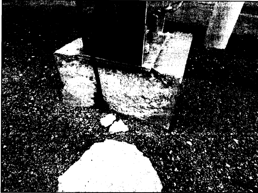
Figure 16: Building 7, Spalled concrete at column pedestal
