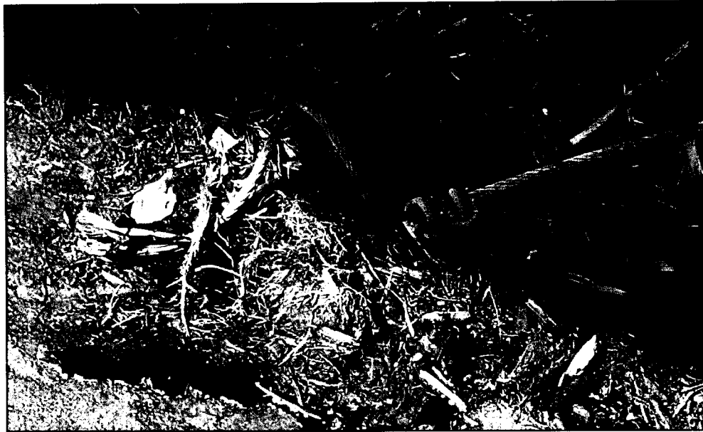
Figure 6: Building 2, Wind bracing cable failure
