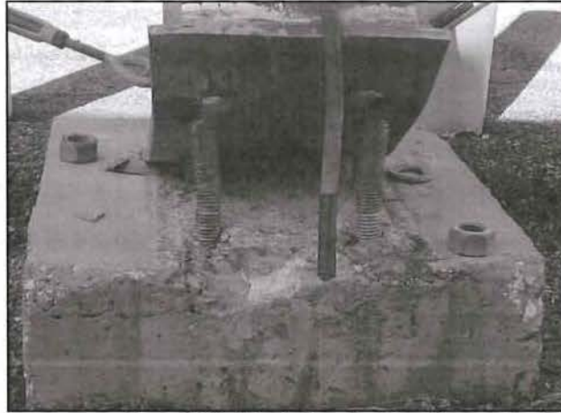
Figure 19: Building 9, Threads stripped from anchor bolt
