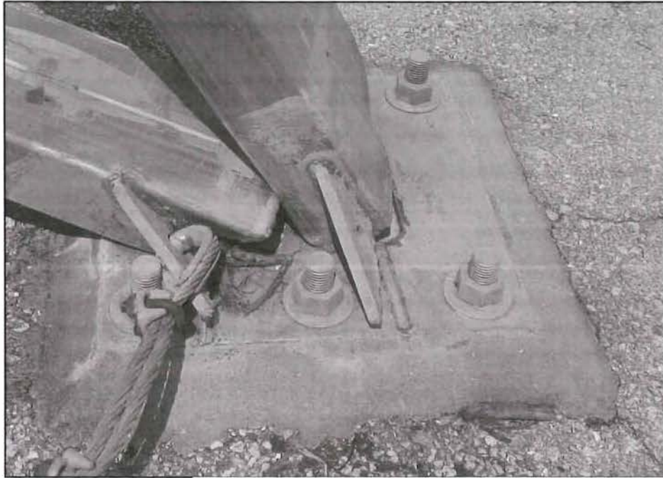
Figure 4: Building 1, Welded joint failure
