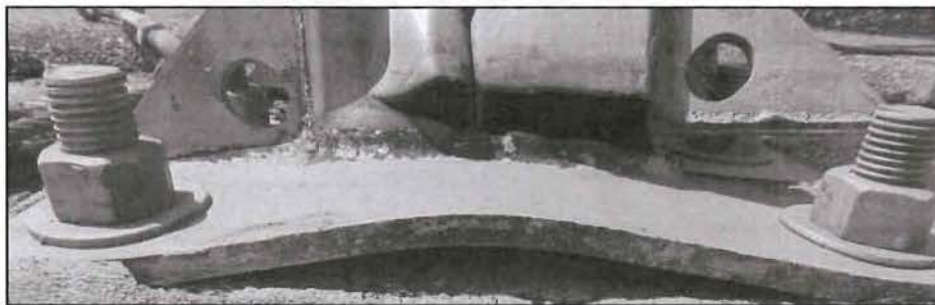
Figure 5: Building 1, Yielding of baseplate
