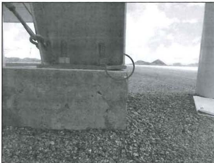
Figure 15: Building 7, Rolled Base plate edge
