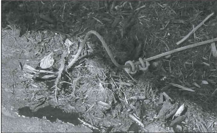
Figure 6: Building 2, Wind bracing cable failure
