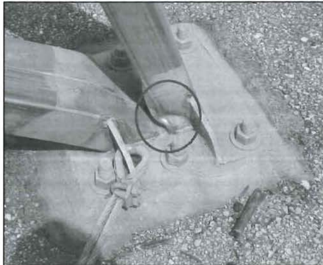
Figure 2: Building 1, Tube sidewall buckling
