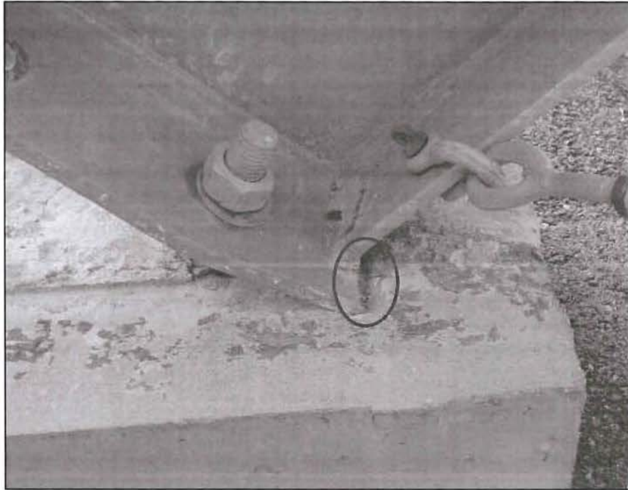
Figure 23: Building 9, Gouging of the concrete pedestal
