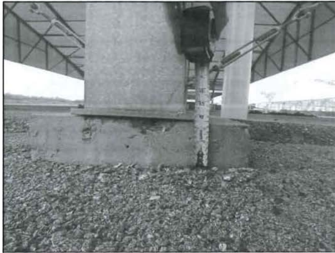
Figure 24: Building 7, Non uniform bearing
