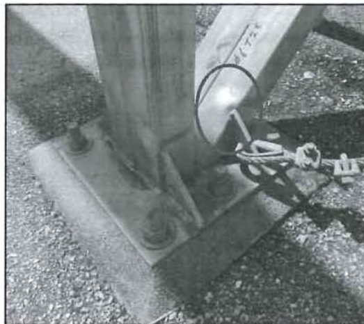
Figure 9: Building 6, Tube wall buckling
