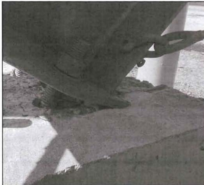
Figure 20: Building 9, Flexure of anchor bolt
