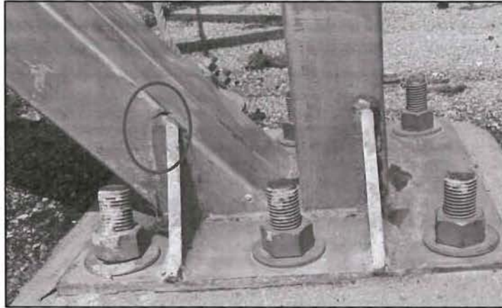
Figure 10: Building 6, Tube wall rupture
