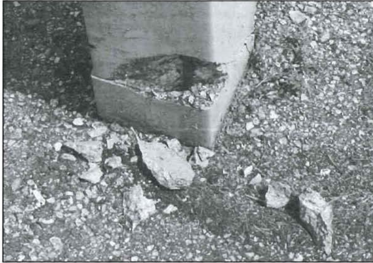
Figure 26: Damaged concrete column
