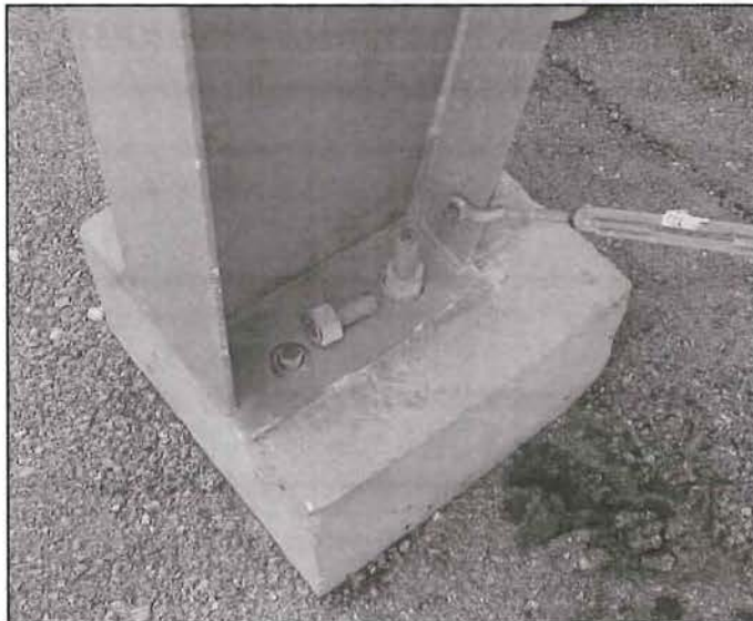
Figure 13: Building 7, Fracturing of anchor bolt
