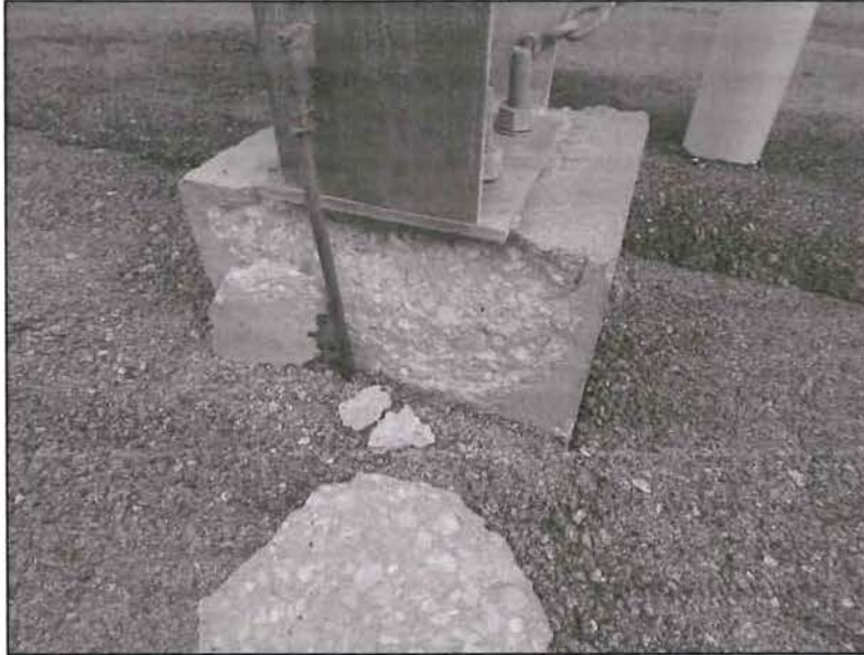
Figure 16: Building 7, Spalled concrete at column pedestal
