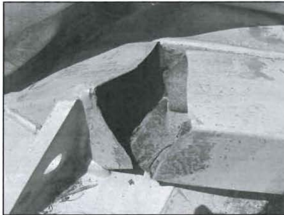
Figure 7: Building 1, Corrosion inside tube
