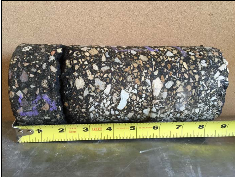
Complete debonding between Lifts 1 and 2.
