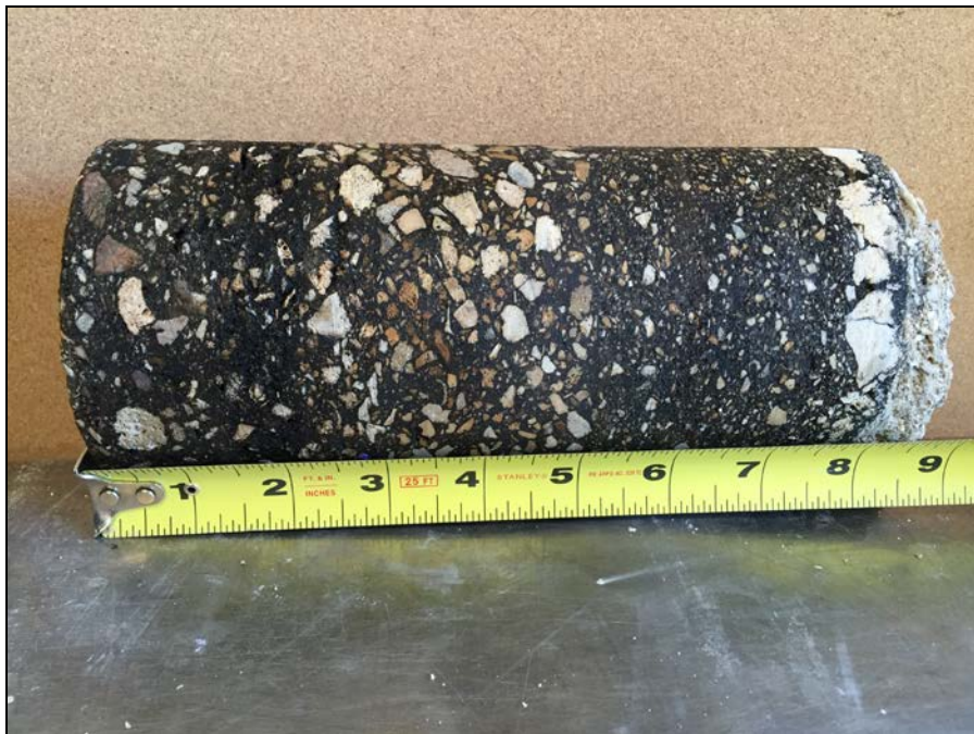
Air voids observed in Lift 2.
