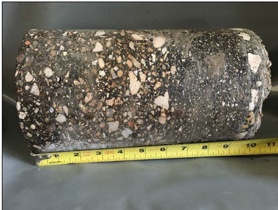
ASPHALT CORE AC-4
