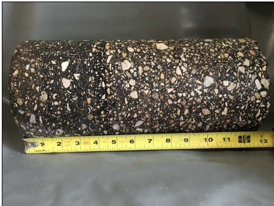
ASPHALT CORE AC-7
