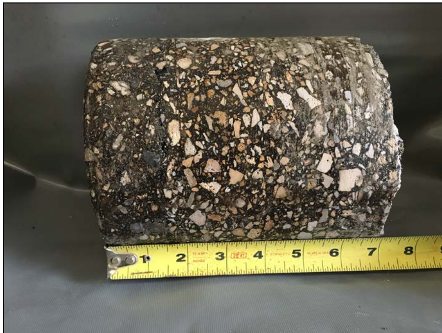
ASPHALT CORE AC-1
